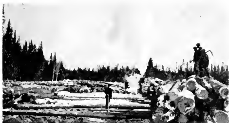
PILING LOGS AT THE LANDING, READY FOR THE DRIVE WHEN THE ICE GOES OUT.
